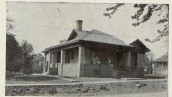
RESIDENCE OF R. W. BRIGGS, LANCASTER, MO.
