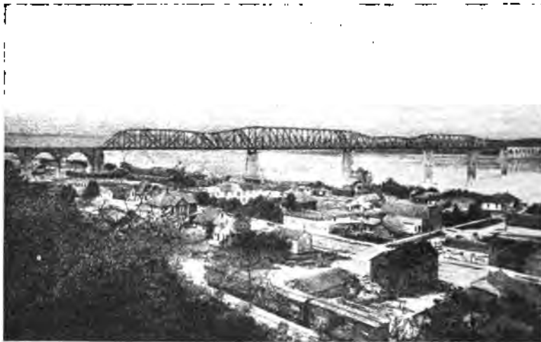
MISSISSIPPI RIVER BRIDGE, THEBES
