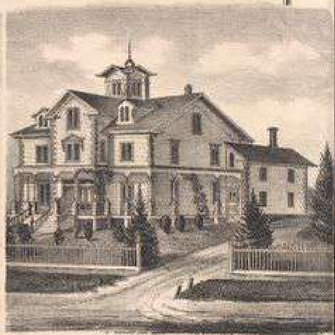
RES. OF F. W. WALKER BRIDGE CONNORIAN 25, N.Y.
