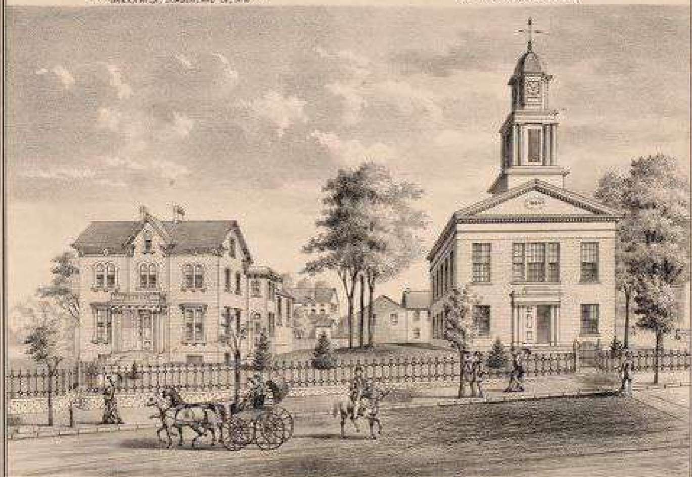
COURT HOUSE, JAIL AND SHERIFFS RESIDENCE, BRIDGEFORD, COMBEE CO., N. J.
