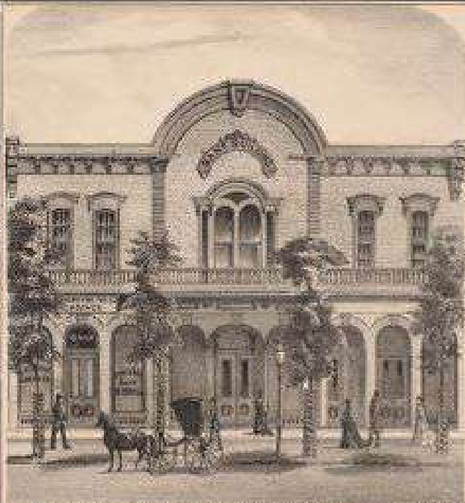
BANKING HOUSE OF THE VINELAND SAFE DEPOSIT COMPANY. DESIGNED BY W. A. HOUSE, PHILADELPHIA. BUILT BY C. W. WOOD, 1880. VINELAND, N. J.
