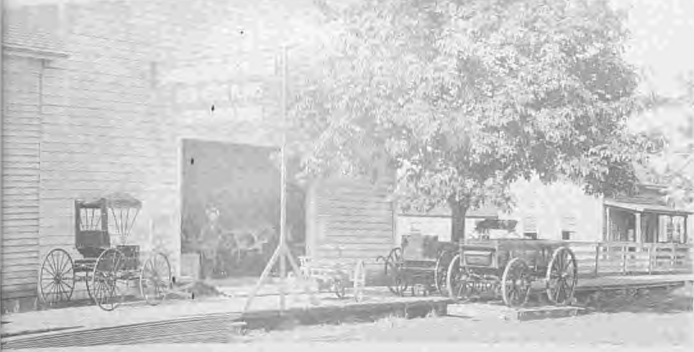
Martin & Sanders Wagon Shop, Court St., Dallas, Ore.
