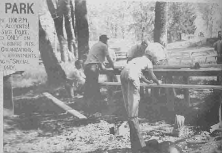
Buell Grange members building benches during park remodeling project.
