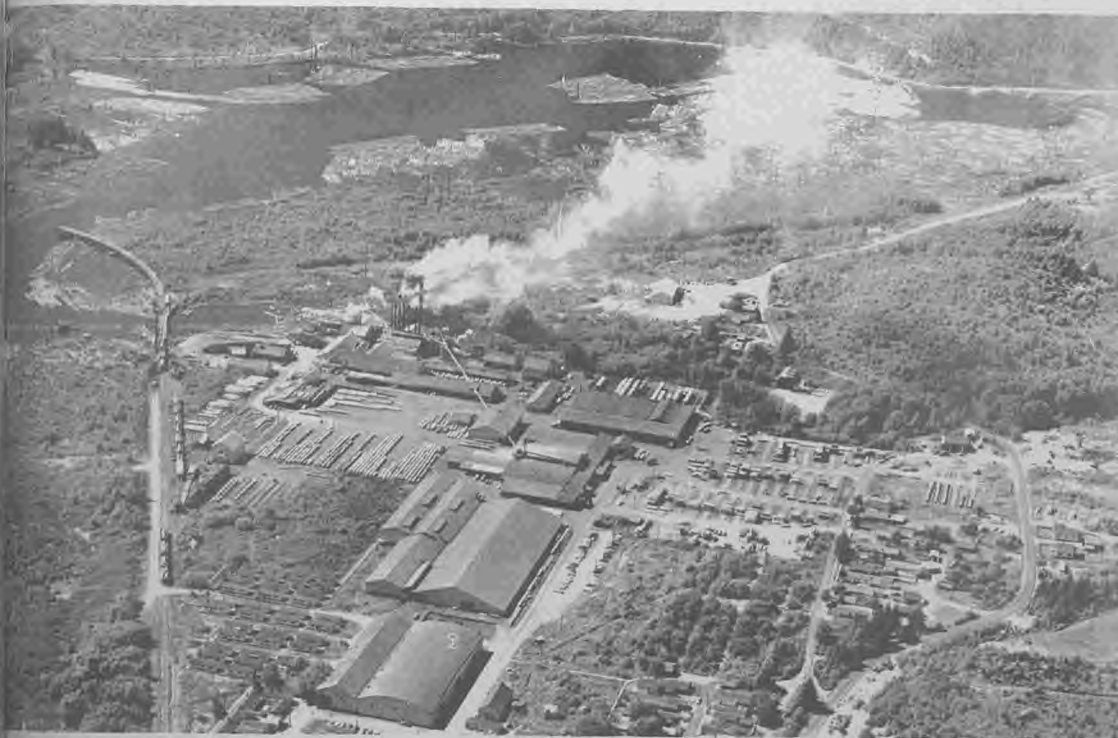
Aerial photo taken in 1955 of Valsetz Lumber mill and log pond also a partial section of town. Log pond covers about 720 acres
