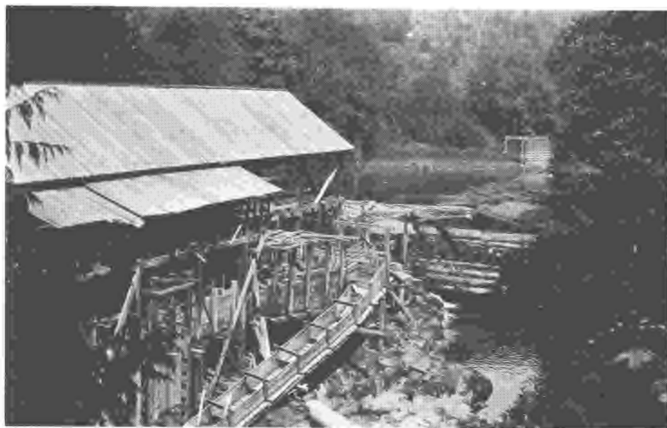
A. C. Reid waterpower sawmill, showing dam and fish ladder. Mill was located a quarter mile below grist mill on Cedar Creek.
