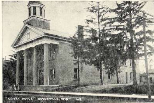
IOWA COUNTY COURT HOUSE, DODGEVILLE, WIS.
