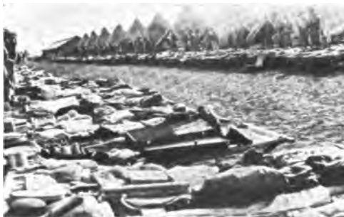
EQUIPMENT LAID OUT FOR INSPECTION
