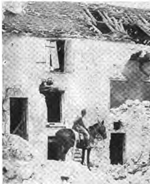
Wrecked building at Chateau-Thierry. The horseman in the foreground is Lt. H. J. Sanders of Racine. The picture was taken July 30, 1919.
