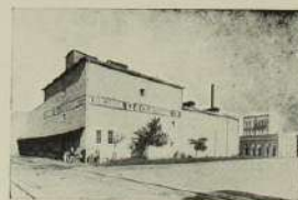
CONCORDIA ICE AND COLD STORAGE COMPANY, CONCORDIA, KANSAS.
