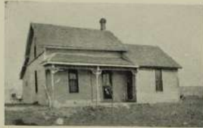
RESIDENCE OF SEVERN CAYER, GLASCO, KANSAS.
