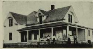
RESIDENCE OF JOSEPH NAILLEUX, R. F. D. No. 4, CONCORDIA, KANSAS.
