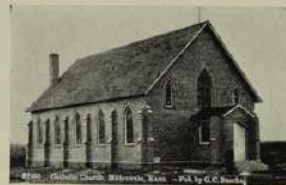
CATHOLIC CHURCH, MILTONVALE, KANSAS.
