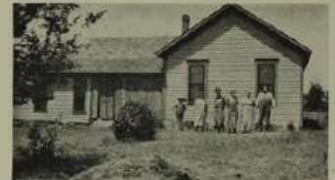
RESIDENCE OF H. F. SMITH, MILTONVALE, KANSAS.
