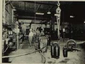
INTERIOR VIEW OF CONCORDIA ELECTRIC LIGHT CO. CONCORDIA, KANSAS.
