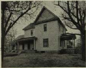
RESIDENCE OF MARTIN CAPPER, AMES, KANSAS.
