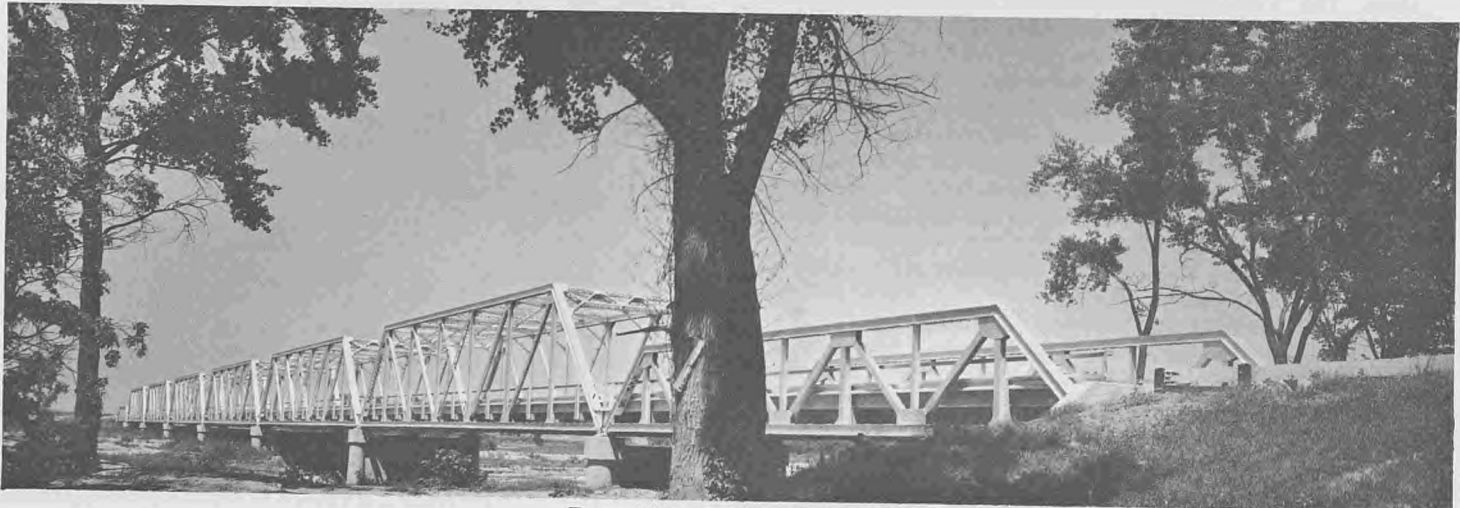
Republican River Bridge
