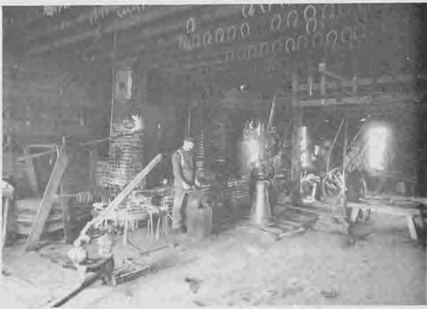
Blacksmith Shop of Charles W. Myers, Corner 6th and State, 1901
