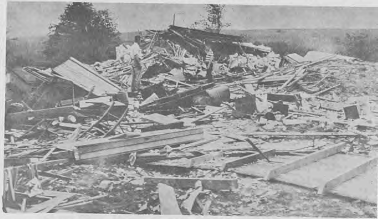
Among the many homes destroyed in the 1957 tornado was the W.E. Keil home, one mile south and two miles west of the KFRM towers. The home was a two story building of limestone.
