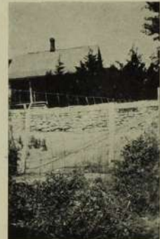
RESIDENCE OF PETER WEDELIN, SEVERY, KANSAS.
