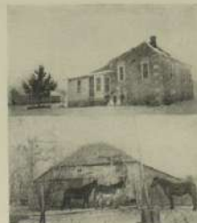
RESIDENCE AND BARN OF AVERY SIMMONS, BAKWARD, KANSAS.
