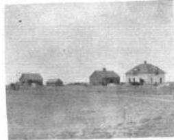
RESIDENCE AND FARM BUILDINGS OF JERRY CORRYELL
