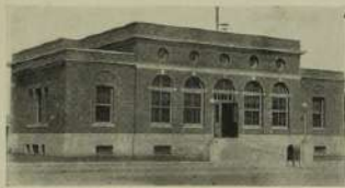
GOVERNMENT BUILDING, OSAGE CITY, KANSAS.
