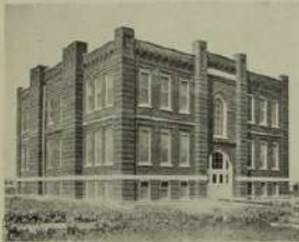
CULVER PUBLIC SCHOOL BUILDING. Photograph from F. G. Brenner, President of School Board, CULVER, KANSAS.
