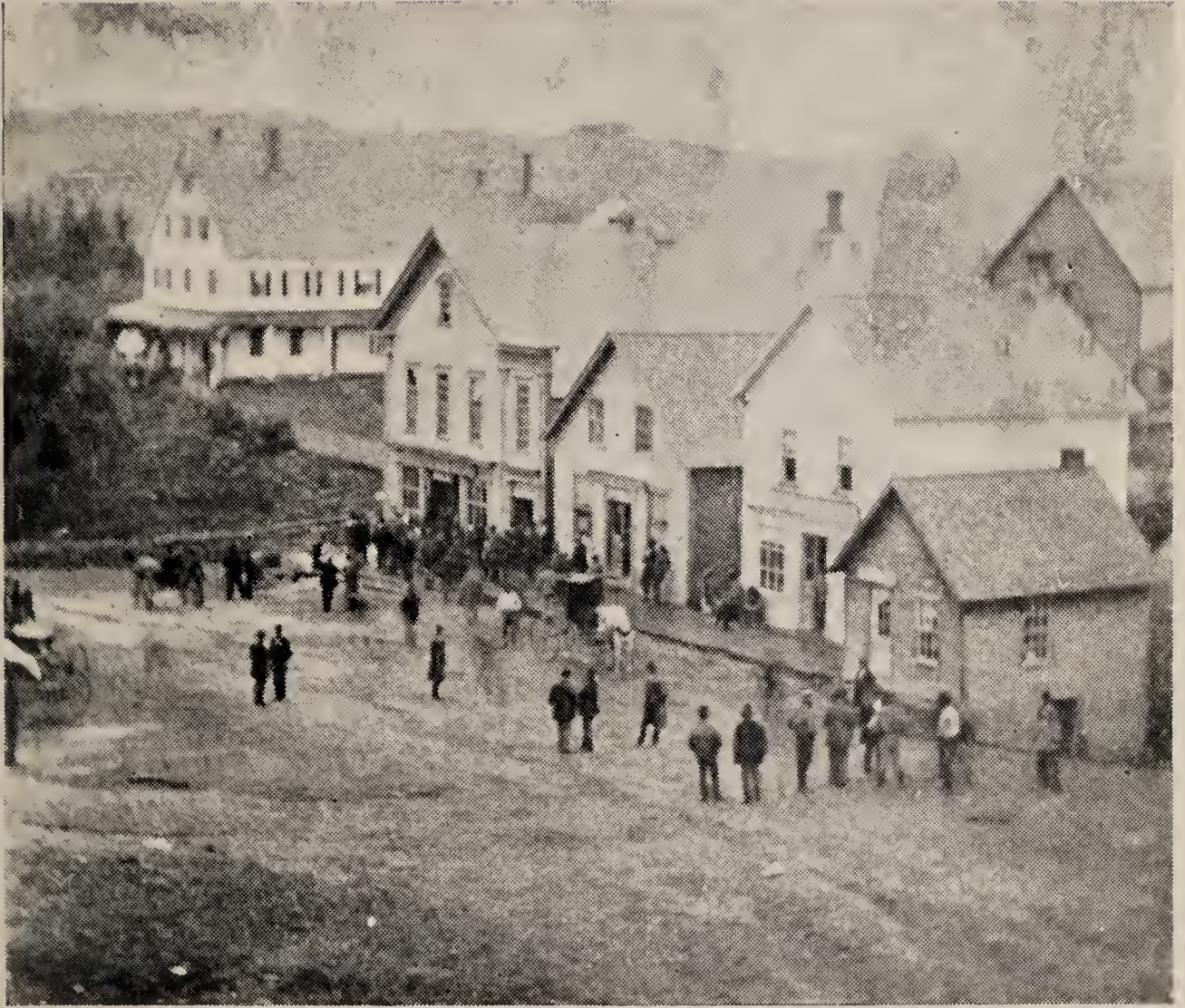
Main Street, looking toward Vaughan House on hill
