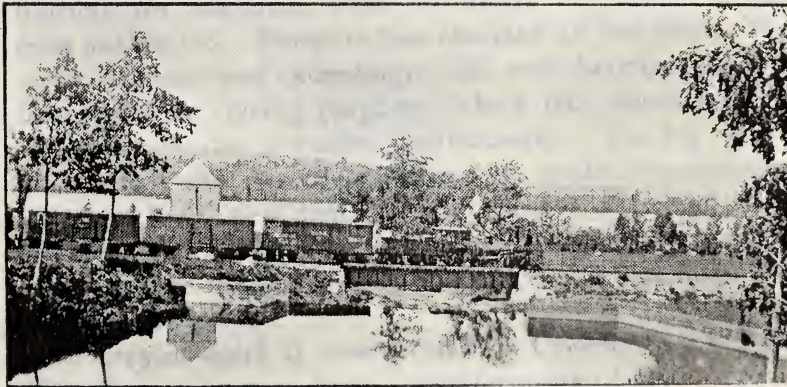
CRAWFORD RIVER, OVERLOOKING THURSTON BROS.' NEW DAM. G. V. R. R. TRAIN ON THE BRIDGE.
