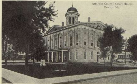
AUDRAIN COUNTY COURT HOUSE, MEXICO, MISSOURI.
