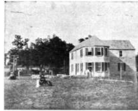
NEW RESIDENCE OF J. H. HOELMER, This building is under construction and is built of solid concrete. HERMANN, MO.
