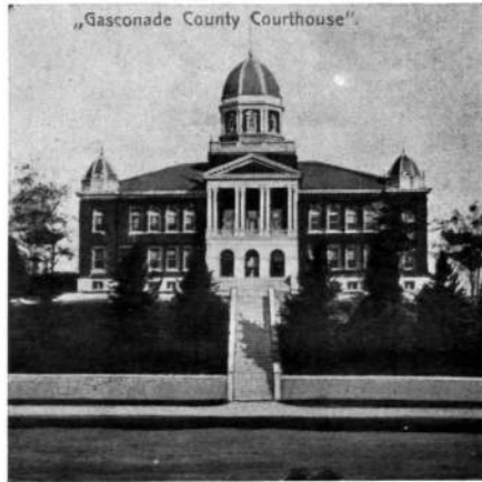
GASCONADE COUNTY COURT HOUSE, HERMANN, MO.
