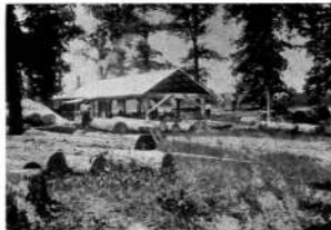
SAWMILL ONE-HALF MILE NORTH OF FREDERICKSBURG, MO. Photograph from Theo. Tegeler.
