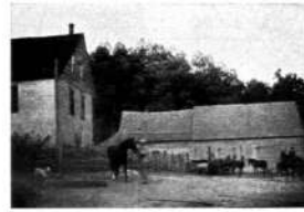
OLD RESIDENCE on the Spring Hill Grain and Stock Farm, owned by J. H. Hoelmer. This house was built in 1847 by Pete Kraetler from sand rocks and red clay. It is very sub- stantially constructed, the walls being two feet thick. HERMANN, MO.
