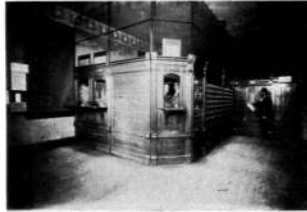
INTERIOR VIEW OF POST OFFICE, HERMANN, MO.
