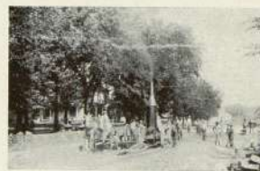
JOHN F. MEEK'S PAVING CREW, Laying Concrete Base on Washington Street, CHILICOTHE, MO.
