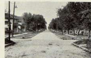
EAST CLAY STREET, CHILlicothe, MO. Paved with "Tarvis" in 1915. Photograph from Harry W. Graham, CHILlicothe, MO.
