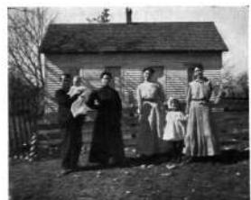
RESIDENCE OF JOHN A. FRANCISCO.
