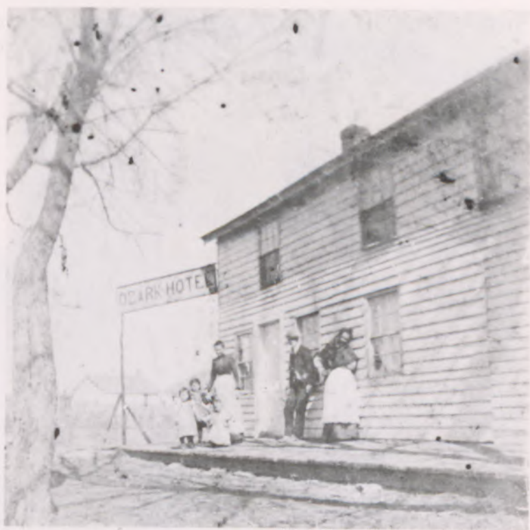
Right, early Ozark Hotel, location unknown. Below, lobby of Ozark Hotel [during 1920's - '30's] located at what is now northwest corner of 8th and Elm.
