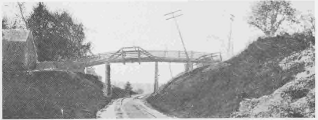
Footbridge over Frisco Railroad track on Main Street between 3rd and 4th Streets.
