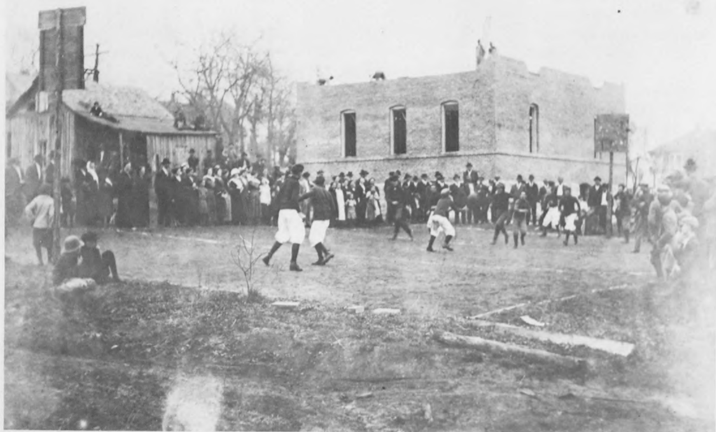
East Elementary School
