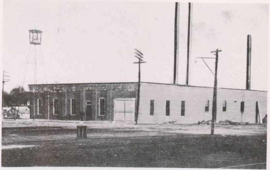
Electric light, power and waterworks plant, 8th Street east of Frisco tracks.
