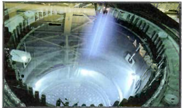
The BLUE Light generated by the irradiated fuel bundle during initial fuel loading
