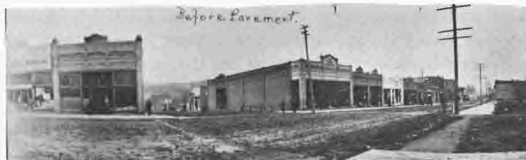
Main Street Before Pavement
