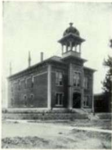
KLUCKITAY COUNTY COURT HOUSE, GOLDENHALL, WASH.
