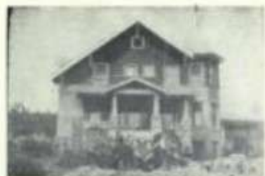
RESIDENCE OF C. K. LARSEN, WHITE SALMON, WASH.
