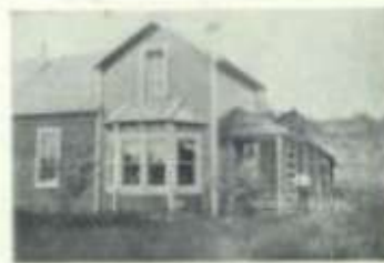
RESIDENCE OF RICHARD J. DODD. BLACKBURN, WASH.
