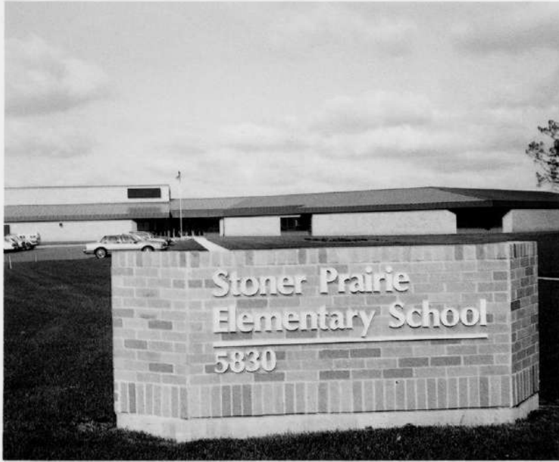
Stoner Prairie Elementary School is located on Devoro Road, near West Lacy Road. The school was built in 1988 on a farm once owned by Moses and Maria Lacy of the Irish Stoner Prairie Settlement. Photo taken in 1992.
