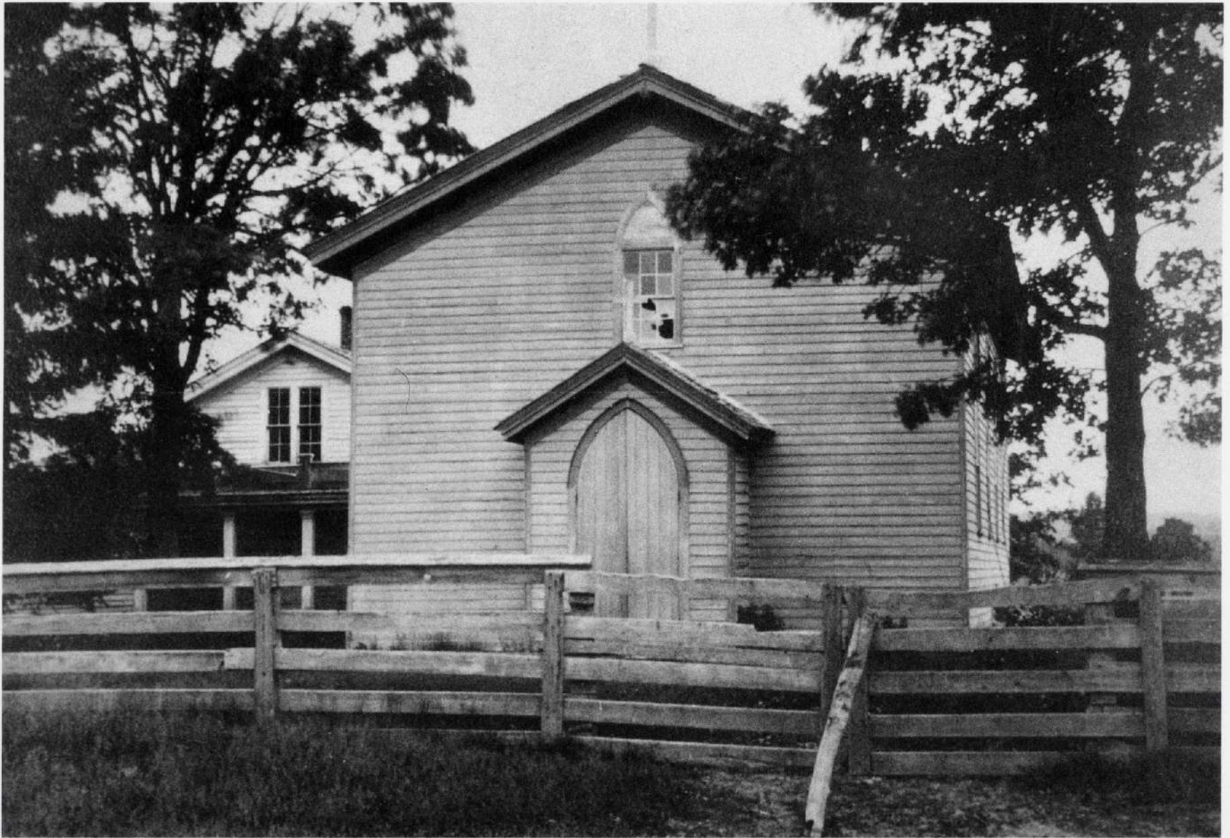
St. Mary's Catholic Church, located west of the gate of the current Oak Hill Correctional Institution on County Highway M, had a large Irish congregation which drew from Fitchburg, Dunn, Rutland, and Oregon townships during the years 1857 to 1886.
