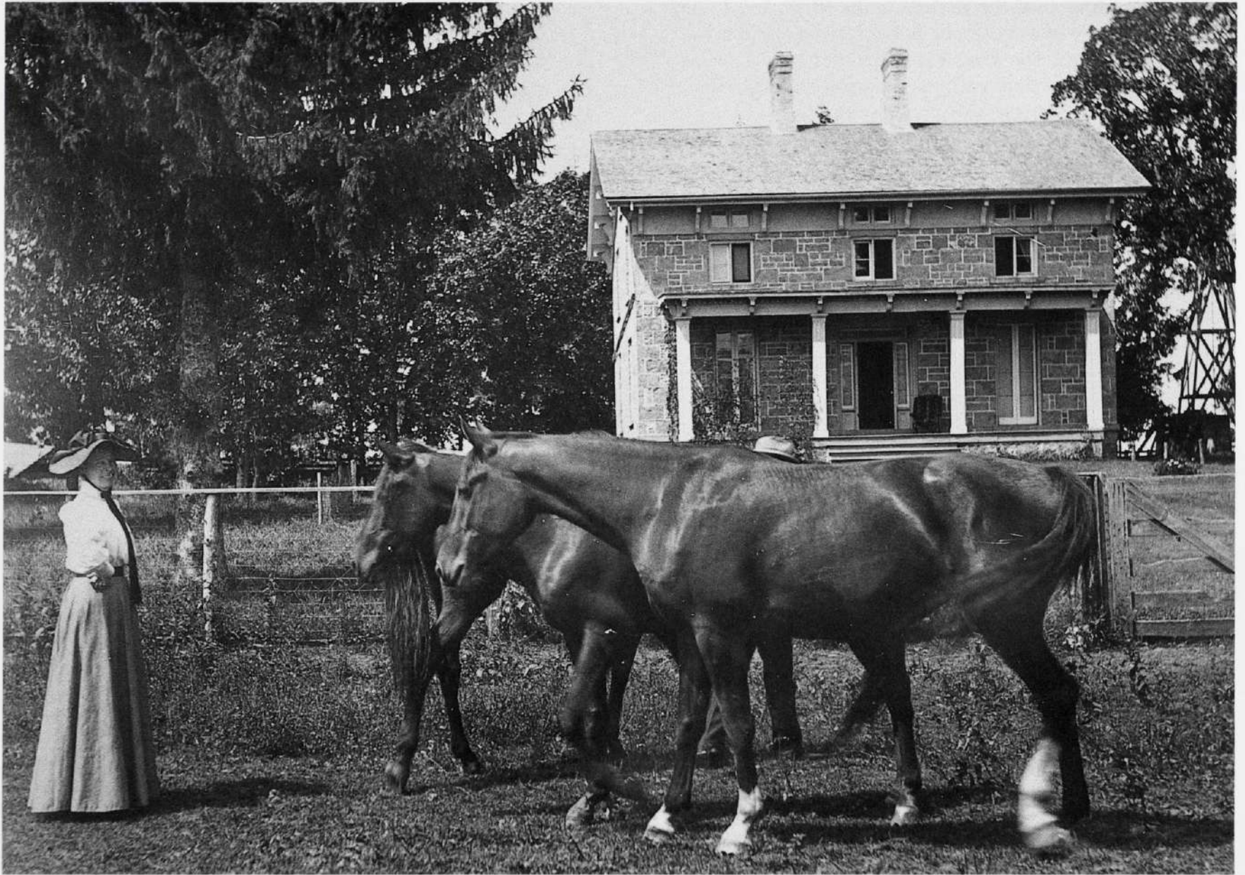
Addie Fox Kiser with horses in front of Fox Hall in 1897. The Italianate house was built in 1856 by George and Catherine Fox from sandstone that was quarried locally and lumber that was transported across Lake Michigan. While the house was being built, the family lived in the basement which had a kitchen and a dining room.
