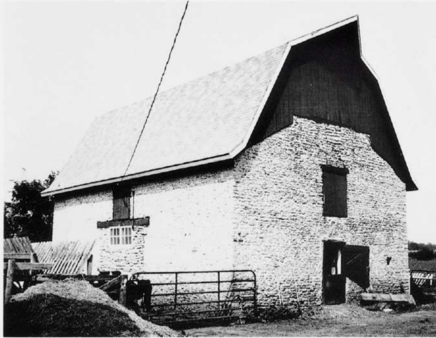
The Martin and Janett McKenna family built this stone barn on their Seminole Highway farm which they purchased in 1856. Note the twentieth century addition of the gambrel roof, which added space to the hayloft. The barn is now owned by Gerald and Ruth Dunn. Photo taken in 1990.
