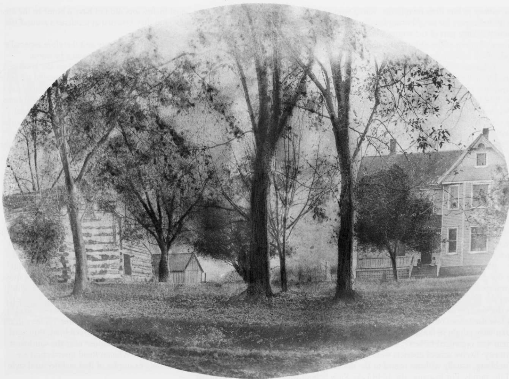
The transition from log cabin to frame house was a welcome event for nineteenth-century pioneers, although the cabin might remain for many years in silent testimony to earlier days. This 1911 photo of the Kinney farm on Irish Lane includes the “upright and wing” frame house with Queen Anne ornamentation that burned in 1920 and was replaced with the present house.
